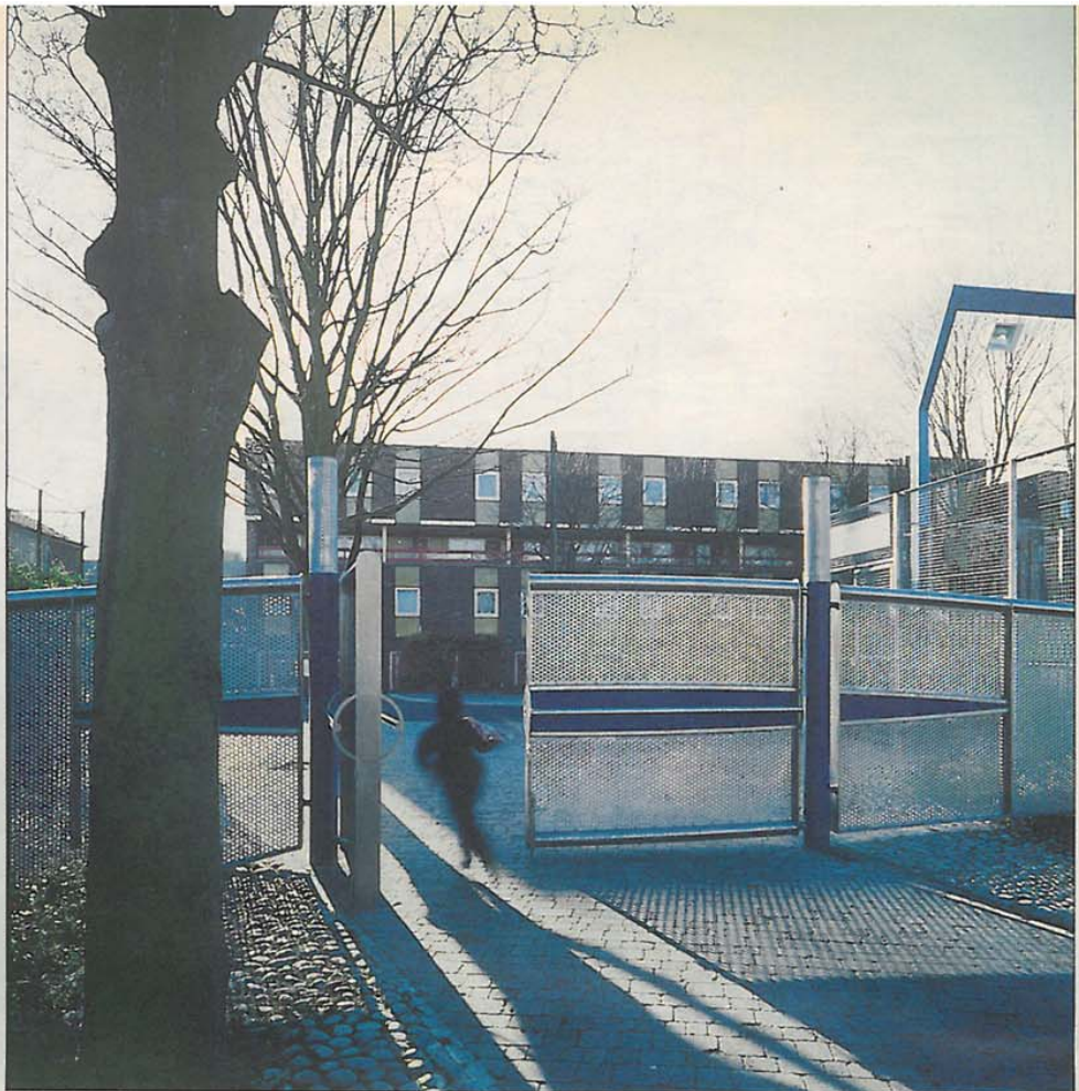
Park life: above, Emslie Horniman Park's perforated stainless steel gate posts, which radiate light from within; and below, the colourful, undulating junior playground
